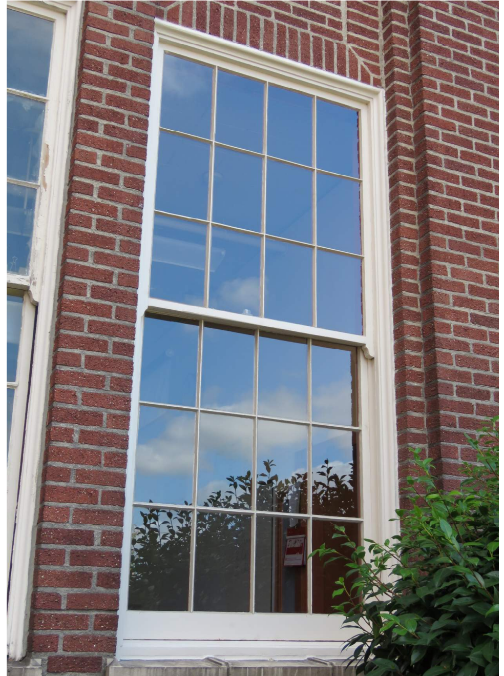
Window E-W-106: After Restoration (Exterior)
