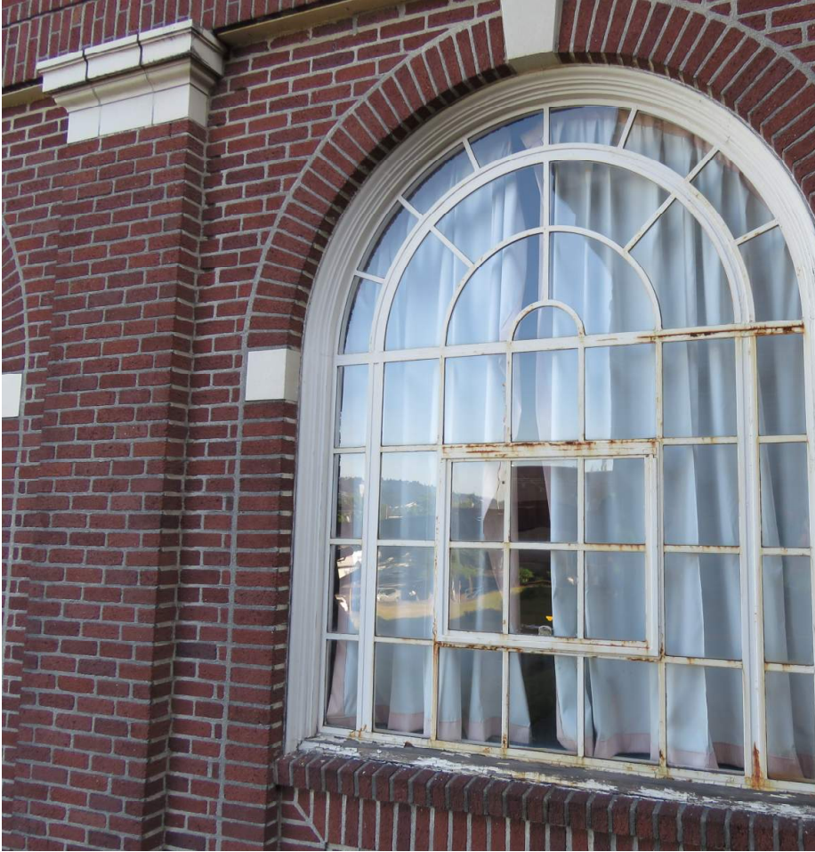
Window A-S-205: Pre-Rehabilitation conditions.
