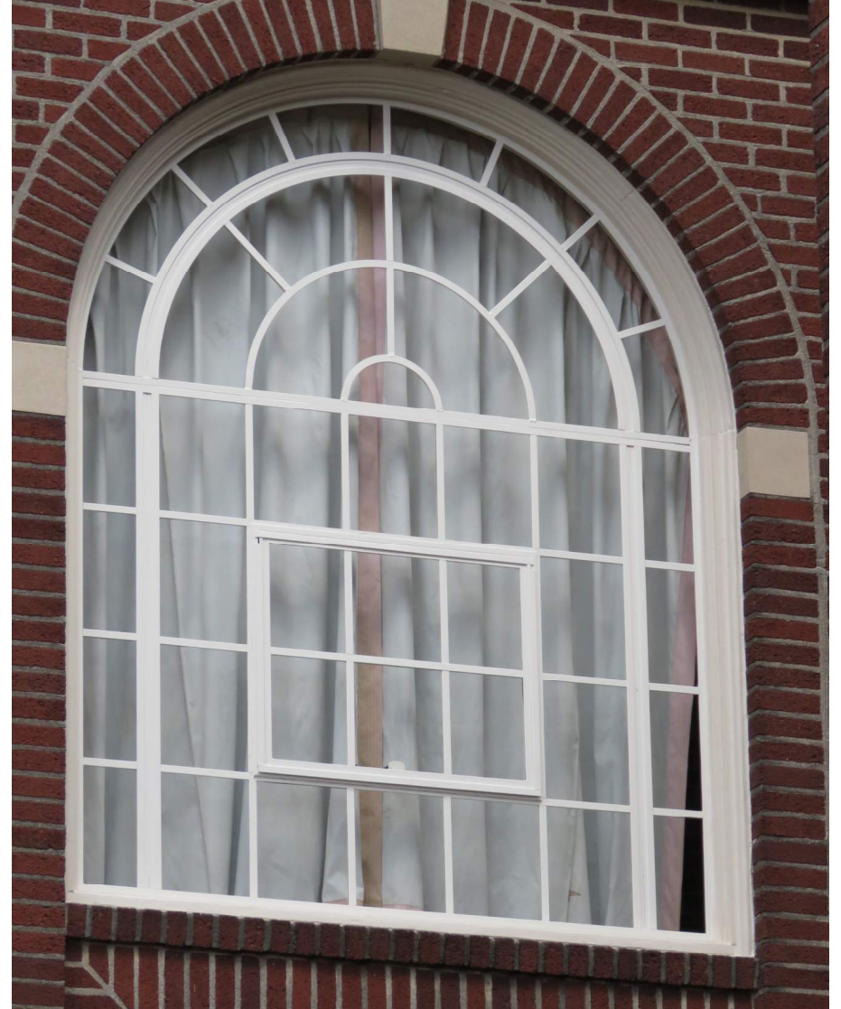
Window A-S-205: After Restoration (Exterior).
