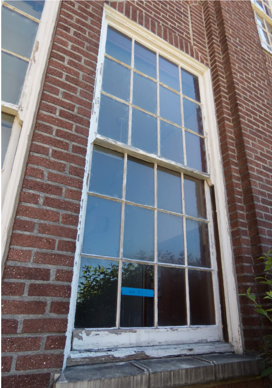
Window E-W-106: Pre-Rehabilitation conditions.
